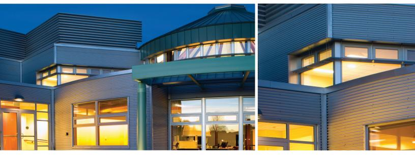
The PBC panels can be used for both roof and wall applications. PBC panels are attached to a building structure with exposed fasteners. The PBC panel is often used in horizontal applications on walls.
